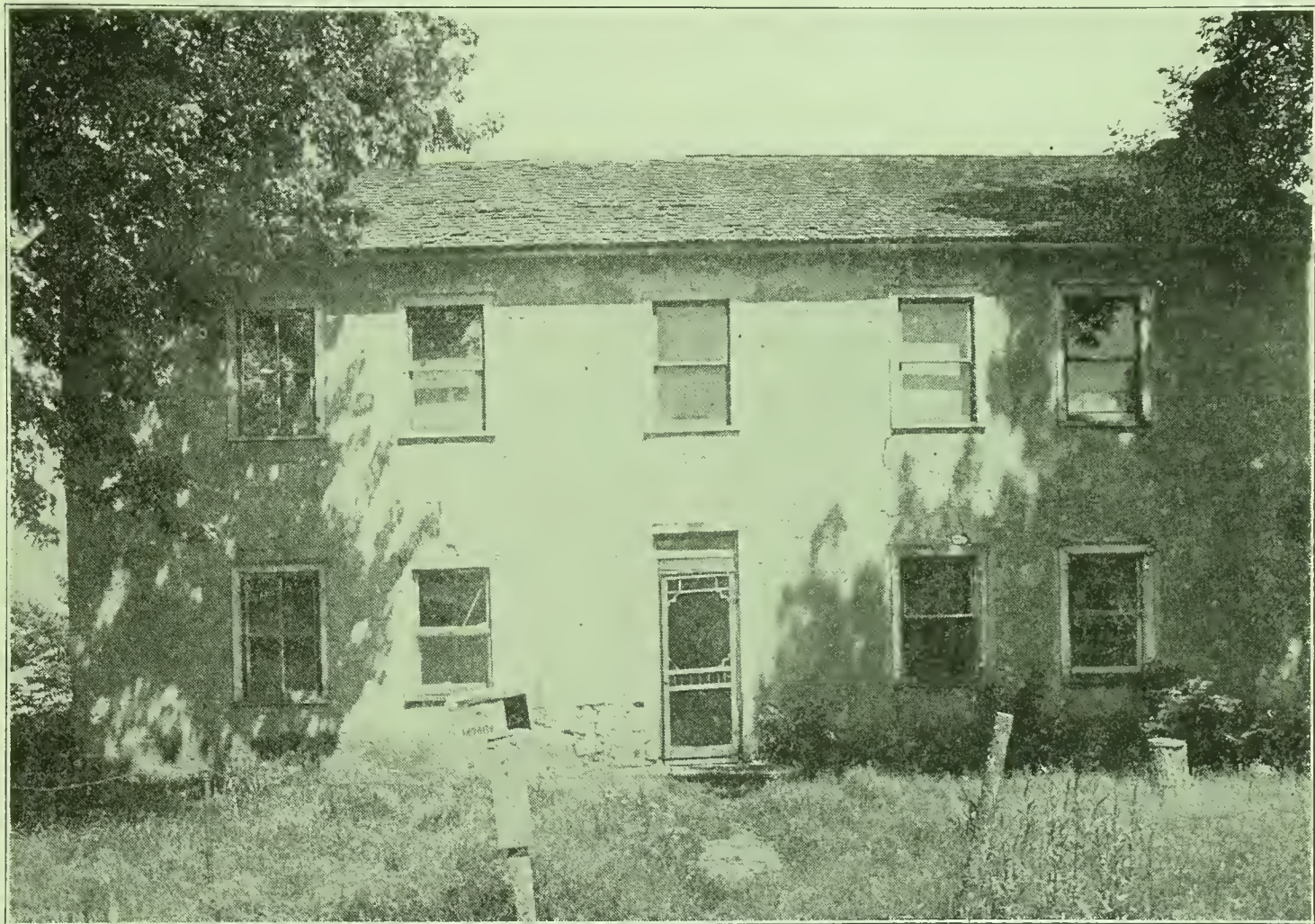
NEBRASKA: PRESBYTERIAN MISSION, BELLEVUE, BUILT IN 1846-47; THE OLDEST BUILDING IN THE STATE
